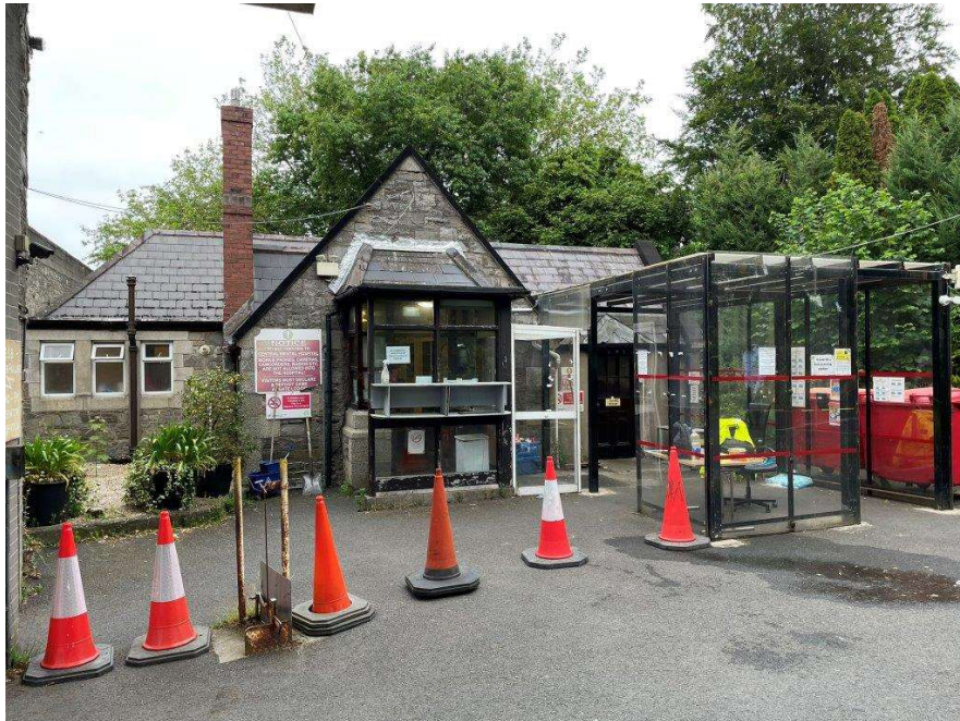
Fig. 04: Southern elevation with temporary structure screening on right hand side
