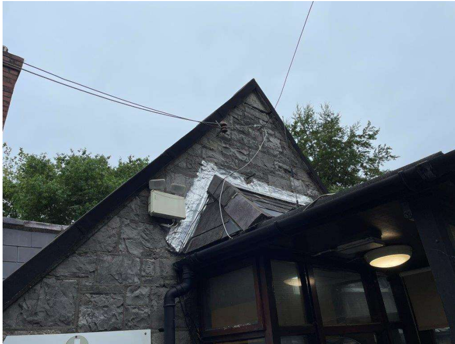
Fig. 08: Flashing where lean-to roof at southern elevation meets stone wall.
