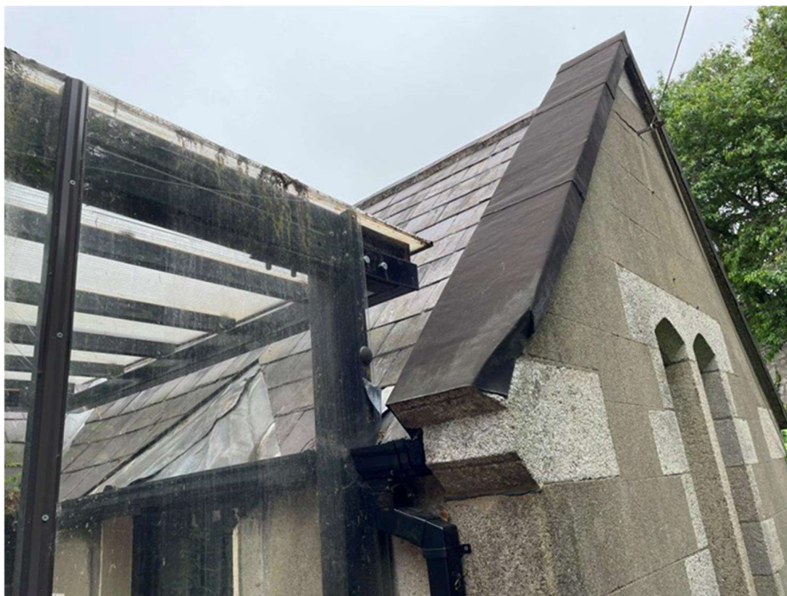
Fig. 05: Junction of temporary screening area and roof of Gate Lodge.
